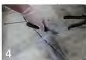
4 Scrape away excess epoxy and smooth surface
