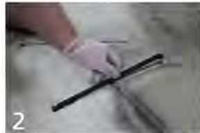
2 Press the CCL into the epoxy
