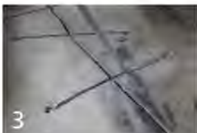
3 Apply additional epoxy over the CCL
